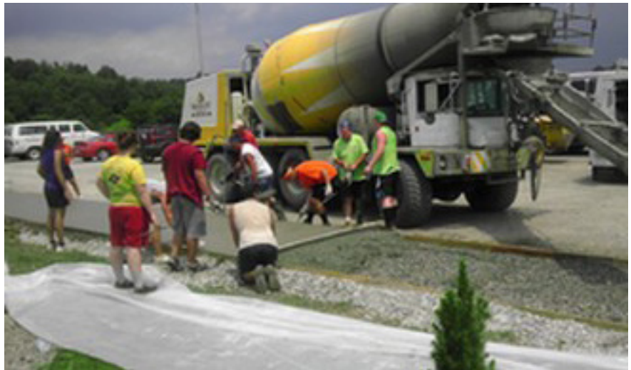
Pictured is the front sidewalk being poured at North Campus
